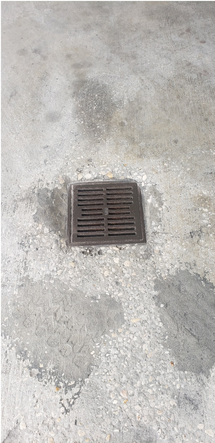
Ramp B landing before main concourse second drain
