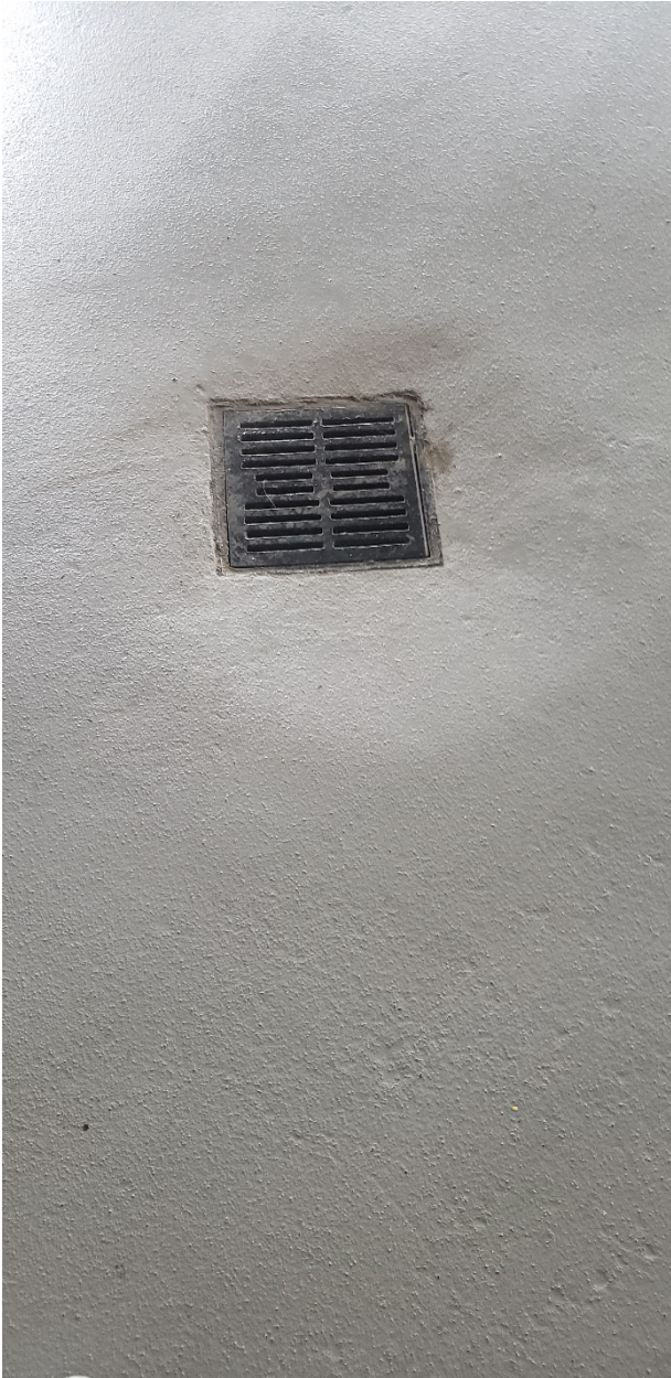
Main concourse in front of B Alcatraz stairs
