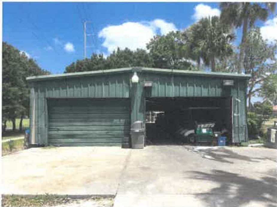
Photo 02 - Rogers Park Golf Course Cart Barn South End
