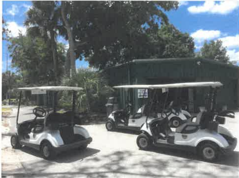
Photo 01 – Rogers Park Golf Course Cart Barn North End
