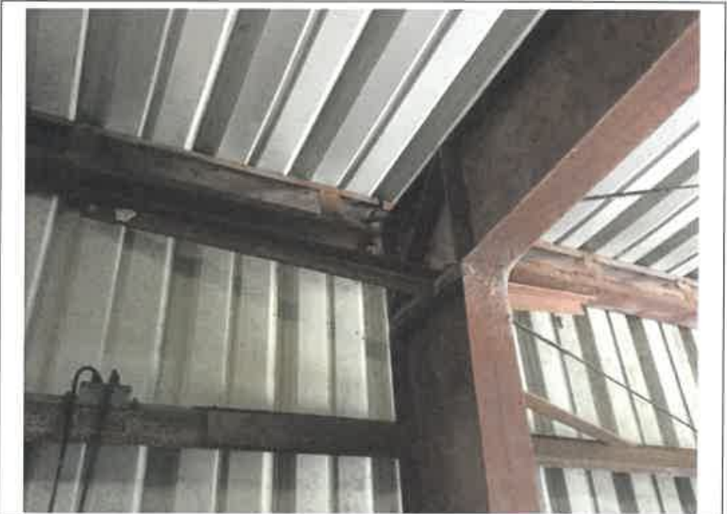
Photo 04 - Rogers Park Golf Course Cart Barn Typical Portal Frame
