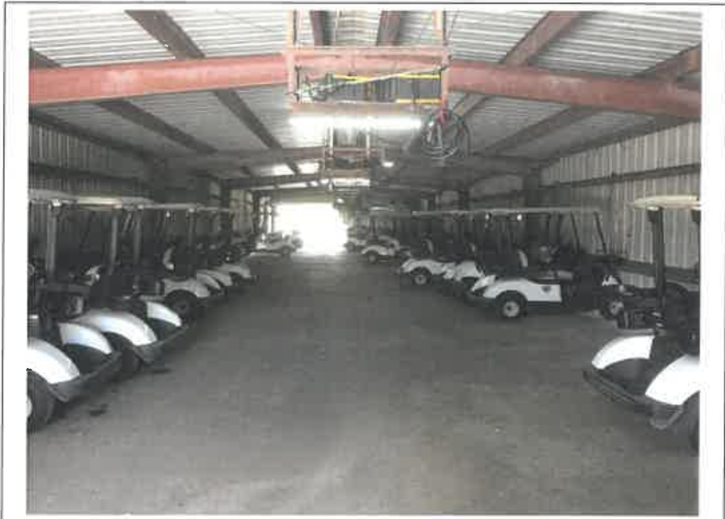
Photo 03 - Rogers Park Golf Course Cart Barn Interior Frame
